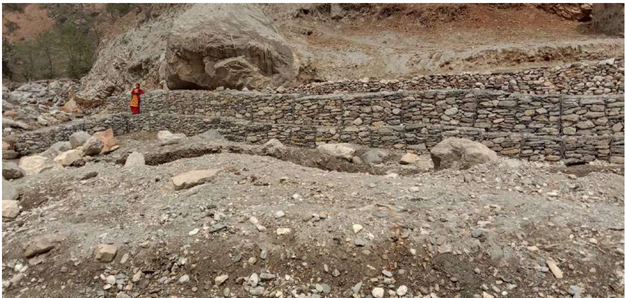
Figure 1: Gabion protection wall construction in Budhinanda#1, Bajedi
