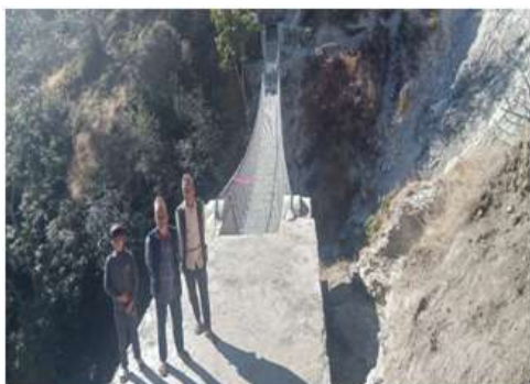
(a) Chunekhola suspension bridge after completion of construction
